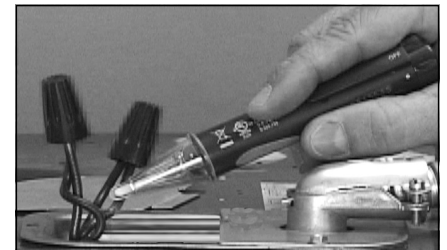
Figure 37 - Non-Contact Circuit Tester
