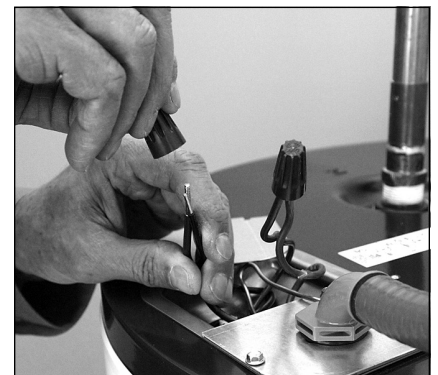
Figure 19 - Connecting the electrical wires.
