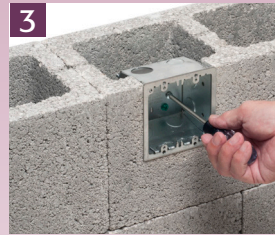
3 Tighten the screws on the spring clip to pull it securely against the block.
