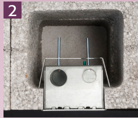
2 Insert the box in the opening in the block. (Top view shown.)
