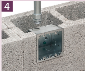
4 Install the EMT in the top of the box.
