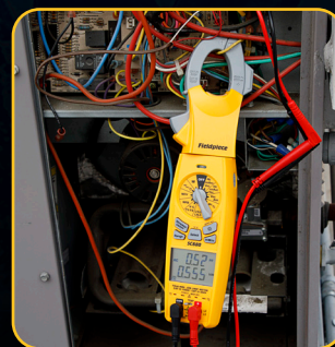
Measures Power (kW)
