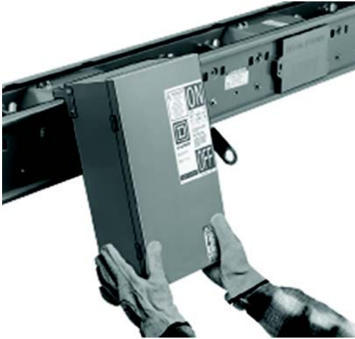
Figure 109: Plug-In Device Mounting
