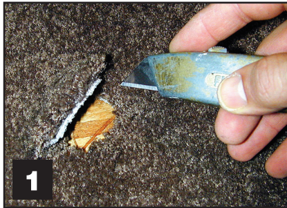
Figure 1 - Cut 2-3/8" hole through carpeting before using a hole saw.
