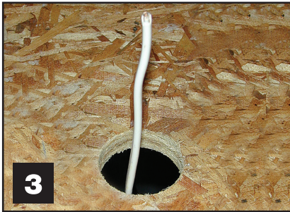
Figure 3 - Pull NM Cable through floor.
