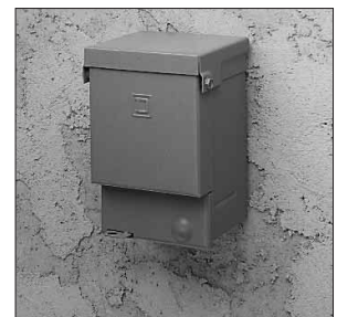
The QO200TR is mounted to the bracket with screws.
