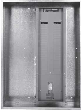
MH38 Enclosure with 6-inch Increased Left-side Gutter
