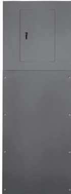
Panel skirt completely installed.
