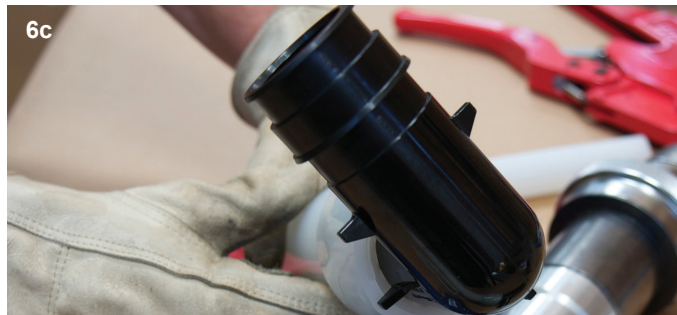
Inserting ProPEX fitting into 2" Uponor PEX piping
