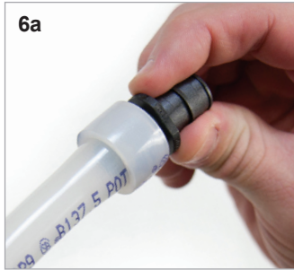
6a Inserting ProPEX fitting into 1/2" Uponor PEX piping
