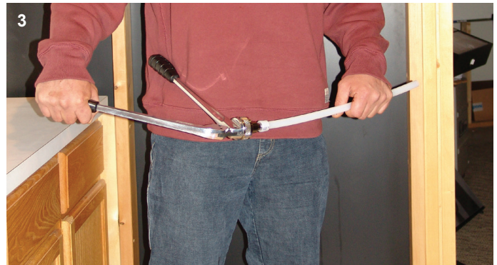
Expansion with ProPEX hand expander tools
