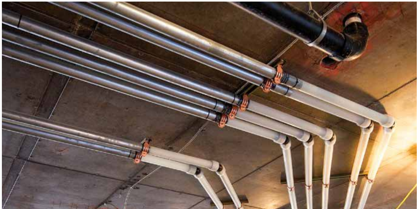
Uponor PEX-a Pipe Support installation at Avalon Bay in Lynwood, Wash.
