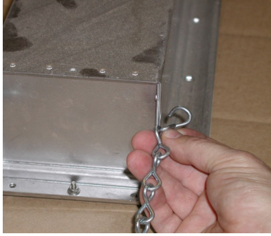
FIGURE 6: ATTACH SUSPENSION HARDWARE
